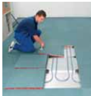
2. Remove at least three adjacent panels.
