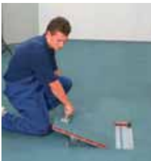
1. Remove panel by lifting device.
