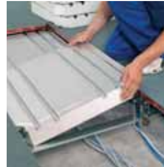
4. Lay in of thermal insulation tray with heat-conductive sheet
