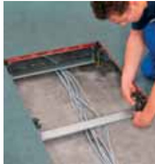
2. Installation of the supporting profiles for the thermal insulation
