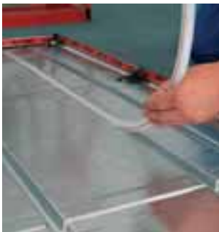
5. Installation of the service lines
