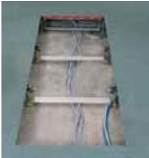
1. Removing of panel rows for the installation of the floor heating/cooling
