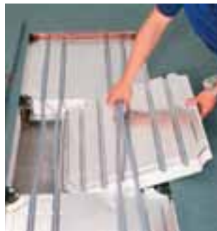
3. Unclip media pipes and hold them up with the spacing device. Take out the insulating tray with transmission sheet by tilting it upwards. Service lines are now accessible.
